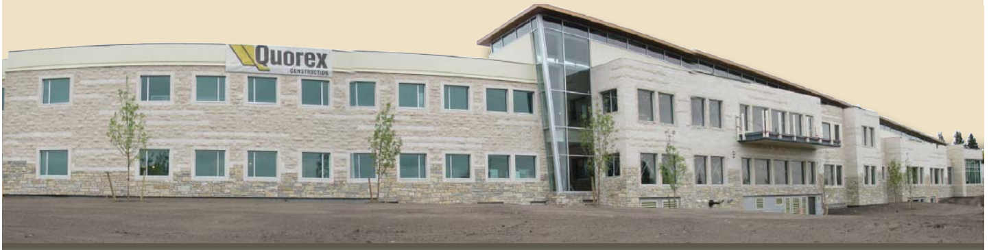
A view of the Irene and Leslie Dubé Centre for Mental Health from the riverbank
